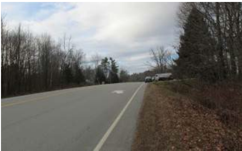
Vassalboro: North Belfast Ave. westbound top end of climbing lane approaching Stone Road intersection.
