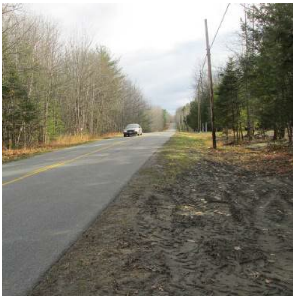
Vassalboro: Bog Road looking west
