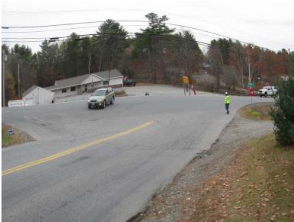
On Summerhaven Road, approach to intersection with Route 27
