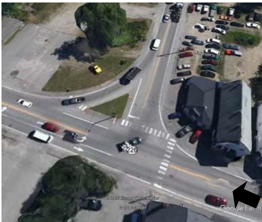
Intersection of Windsor Street (to top) with Water Street (left to right) in Randolph. (Image: Google Earth)
