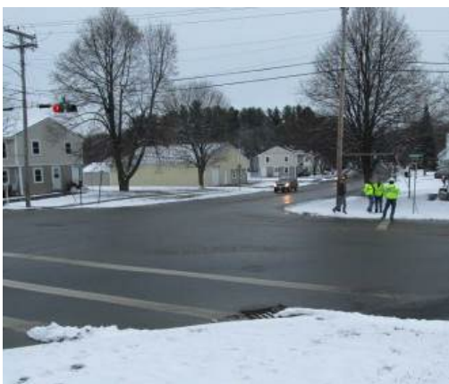
Waterville: Drummond Street (foreground) looking towards Hazelwood, with STOP bar too far back
