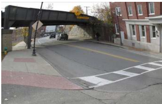
Augusta: Midblock crosswalk north of underpass
